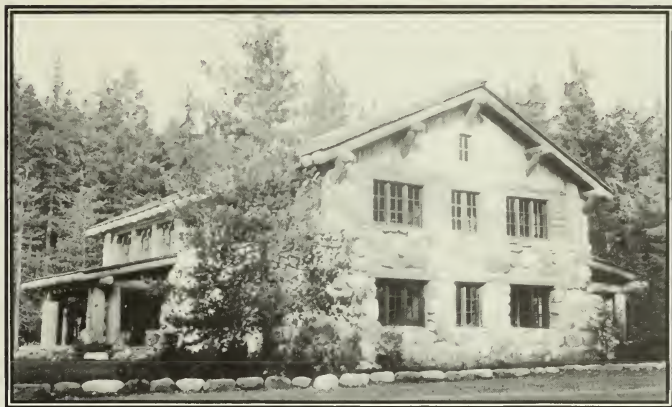
By October 1928 the Administration Building at Longmire was completed. The project took five and a half months with a cost of $3.40 a square foot of floor space. The result is indeed the "very striking structure" the planners intended. (Park Structures Collection)
